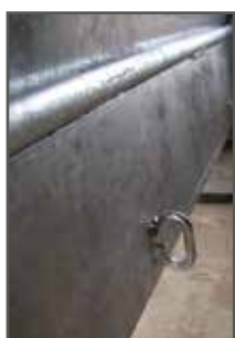
chain links welded on
