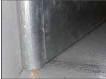
side cleaning flap attention: sharp edges! (-> round off!)
