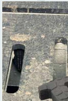
*The individual mats are installed without screwing them to the floor. The studs are knocked in with a hammer to hold the mats in place and prevent them moving sideways on the floor. Matching studs are supplied with the mats.*
