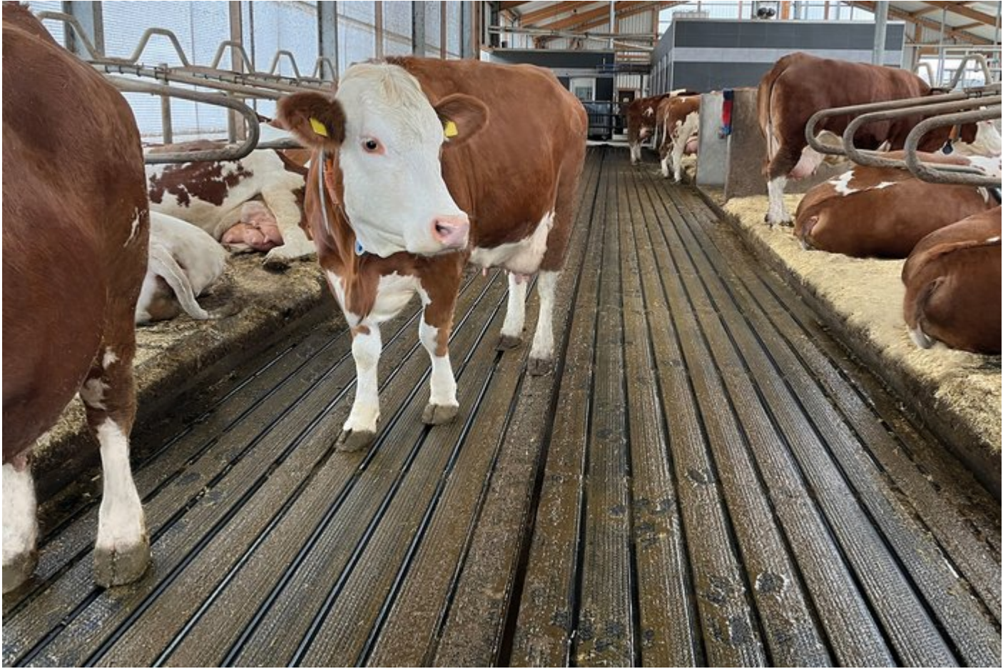
The profiDRAIN drain channel mat combines walking comfort with reduced emissions © KRAIBURG Elastik
