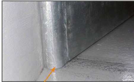
Side cleaning flap Attention: Sharp edges! (-> round off!)
